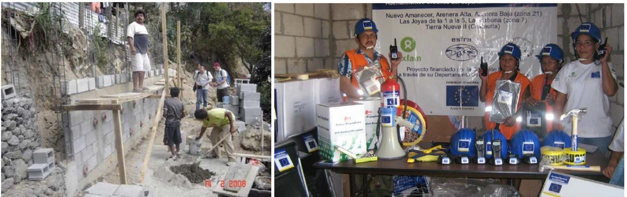
Figure: Support for community-based landslide risk reduction in RiskCity. Left: simple retaining walls are constructed by the local inhabitants with building materials supplied by the NGO. Right: equipment donated by the NGO for local landslide risk management: rain gauges, communication equipment etc.
